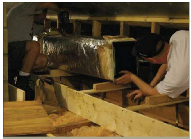
FIGURE I-12 Duct insulation increases system energy efficiency.
