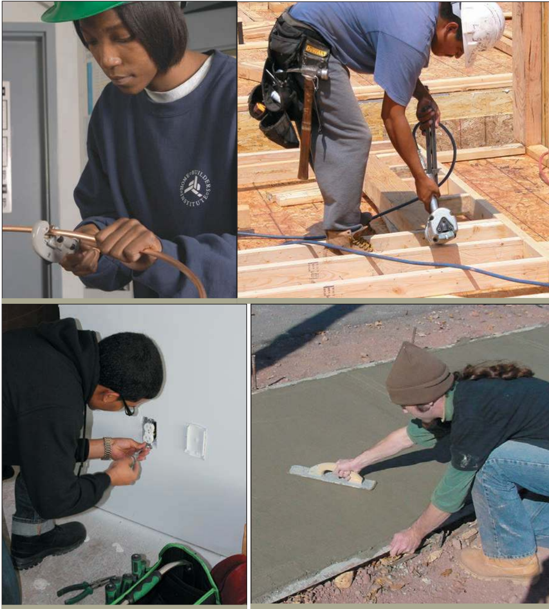
FIGURE I-10 Work on the job requires cooperative efforts by different individuals from different trade areas.
