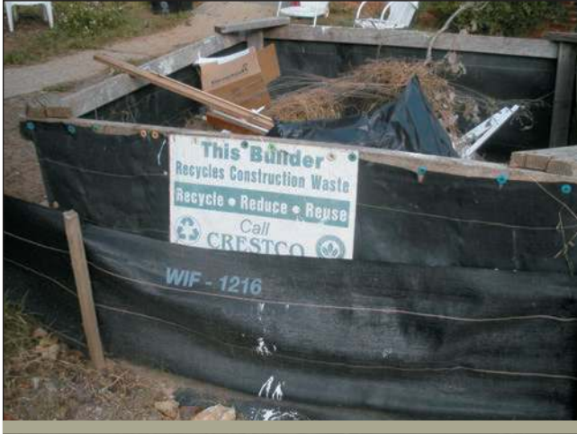
FIGURE I-13 Construction site waste recycling. Courtesy of Carl Seville.
