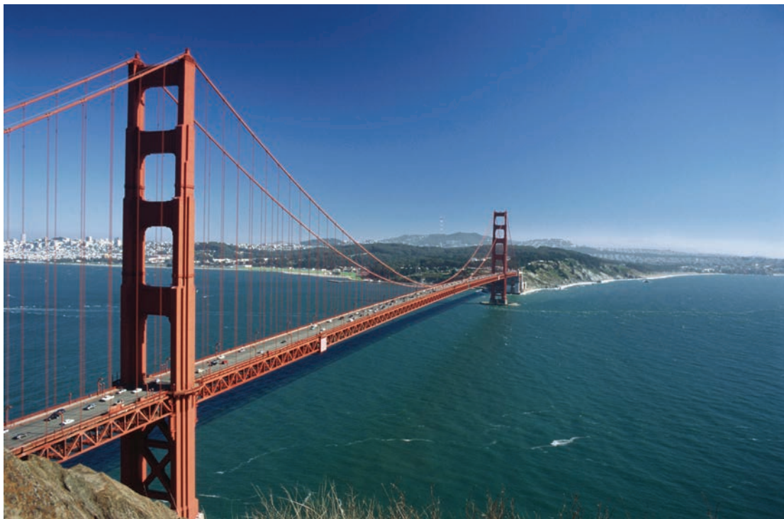
FIGURE 1.2 The Golden Gate Bridge north of San Francisco, California, is one of the most famous and most beautiful examples of a steel bridge. (© LOOK Die Bildagentur der Fotografen GmbH / Alamy.)
