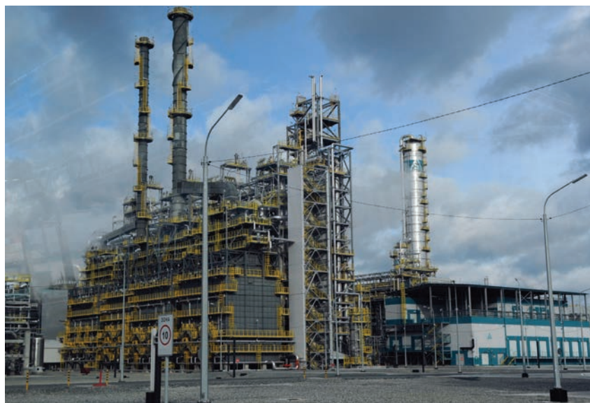
Figure 1.9 Polypropylene plant. Plastics are the substances produced in the greatest quantity by the chemical industry. This plastic manufacturing facility is located in Tobolsk, Russia (a historic capital of Siberia).
