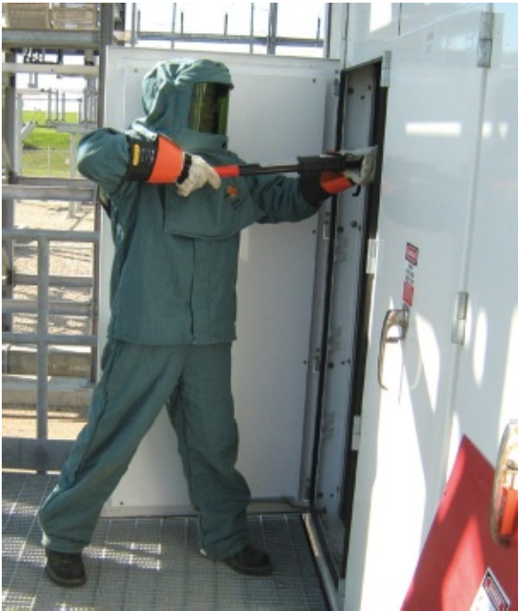
Figure 1-4 An arc flash hazard exists when a person interacts with equipment.
