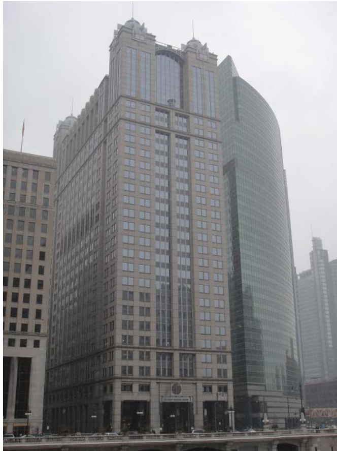
Figure 1-5 The 225 West Wacker building in Chicago, USA (Photo provided by Xiaojian Gao)
